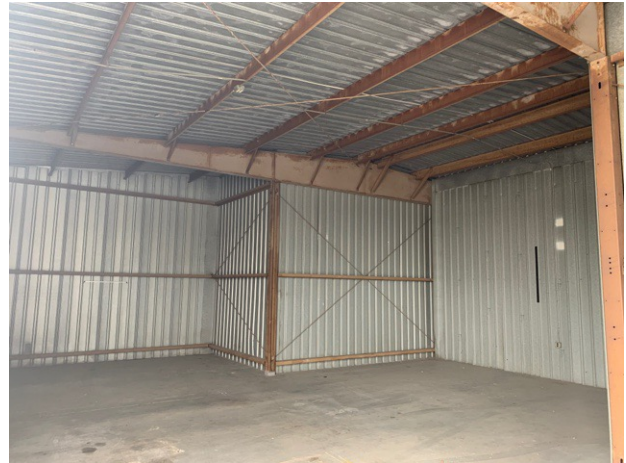
T- Hangar Row S
