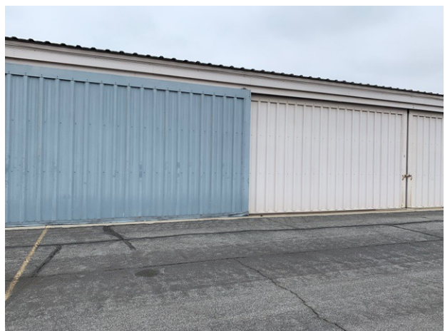
T- Hangar Row S
