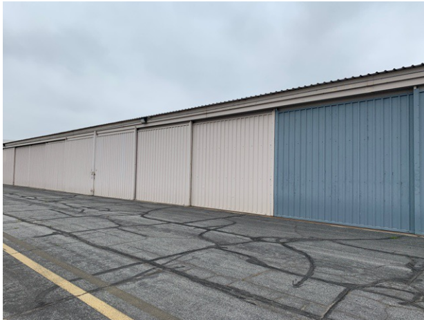
T- Hangar Row S
