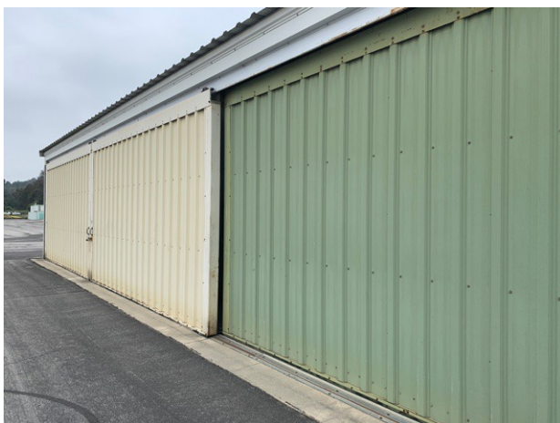
T- Hangar Row J
